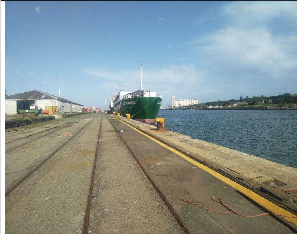
Figure 2: Middle section of the quay
