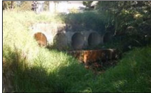
Figure 6: Image of existing bridge
