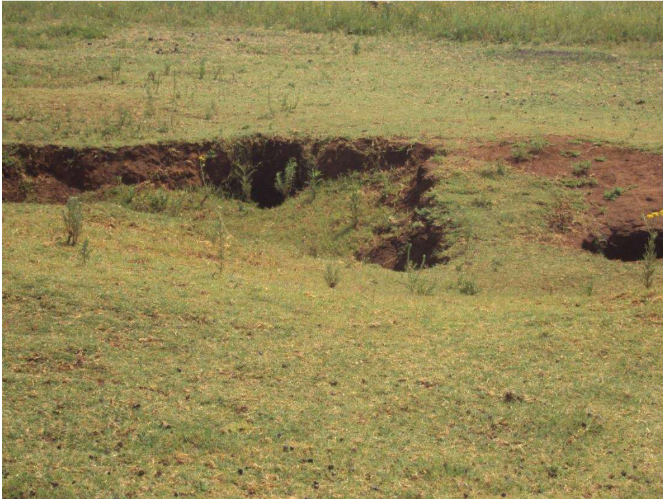
Figure 8: View of sinkhole with animal burrow in the western section of the project footprint
