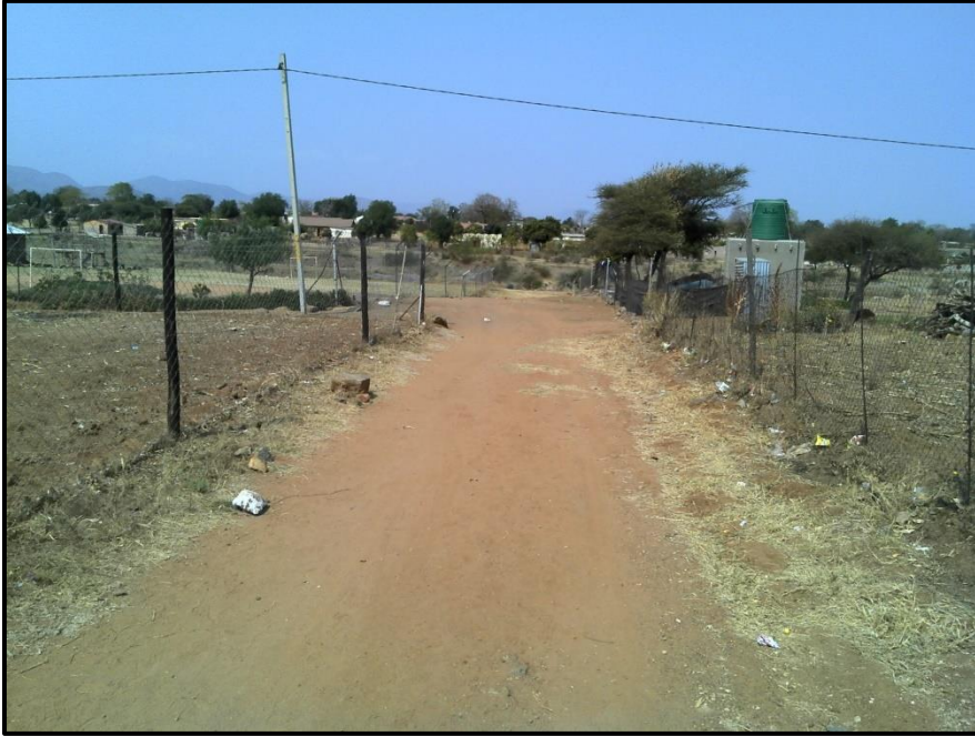
Figure 6. Existing roads, white stones mark pipeline.
