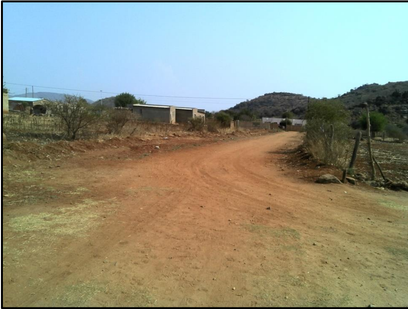
Figure 4. Existing roads that the pipeline follows in Ga-Mapela.
