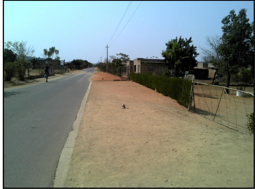
Figure 7: Road reserve that the proposed pipeline follows.
