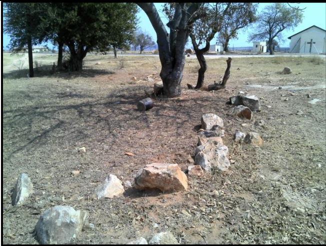
Figure 8: Remains of Stone Wall foundation.
