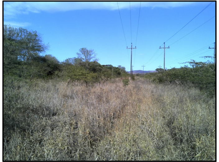
Figure 5. Existing power line corridor.
