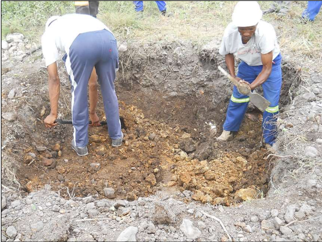
Figure 4. Digging deeper into rock-bottom.
