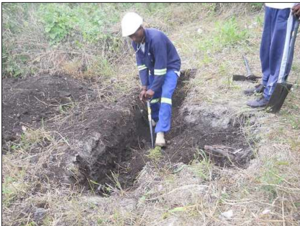
Figure 8. The excavated test trench and beginning of the extension at Shazi 2 grave.
