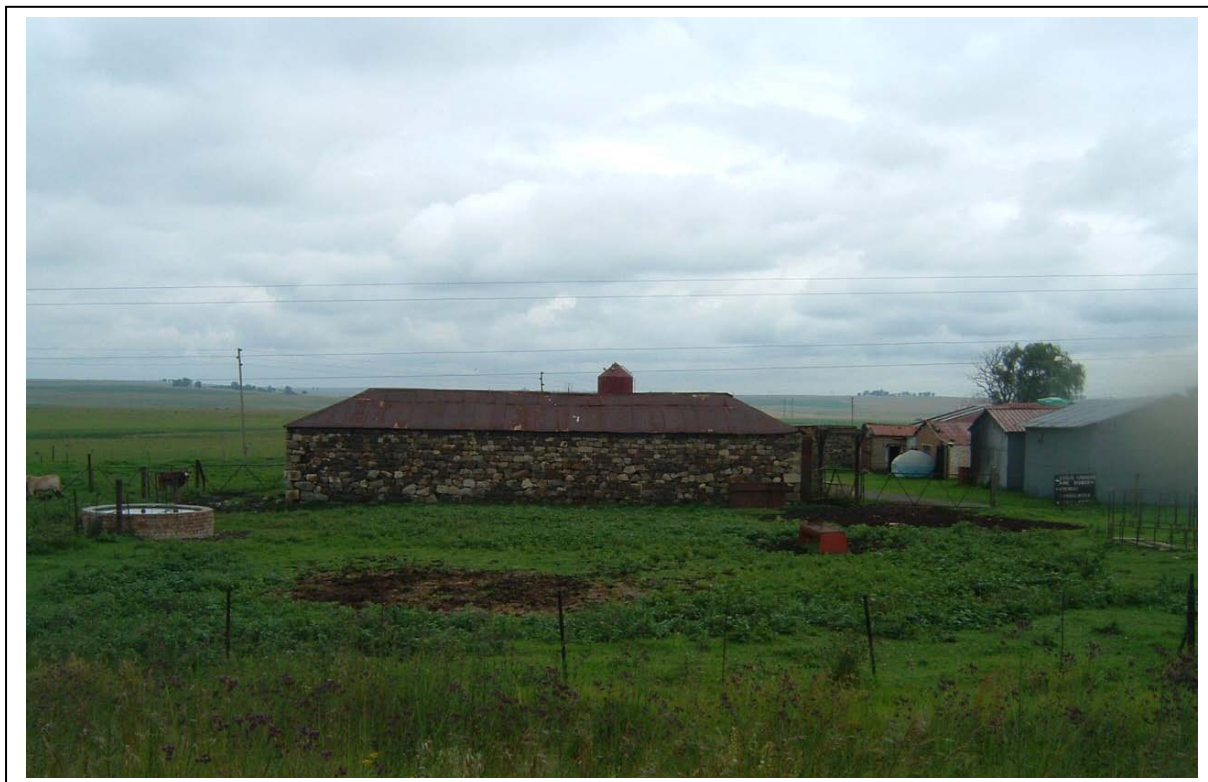
Figure 10- A wagon shed constructed with sandstone on Rietkuil 531IR next to the Leandra-Balfour road (above).
