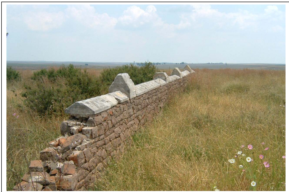
Figure 23- The wall that demarcates GY20 is constructed with dolerite stone and capped with sandstone trimmings (above).
