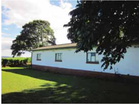
Fig 30: Edge from the access road
