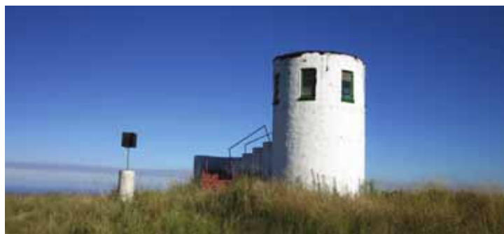
Fig 32: Fire Lookout tower
