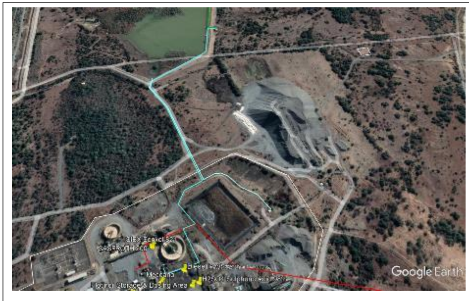
Figure 12- Both these short pipelines (light blue) follow the shoulder of a haul road one entering the Meccano Plant (above).
