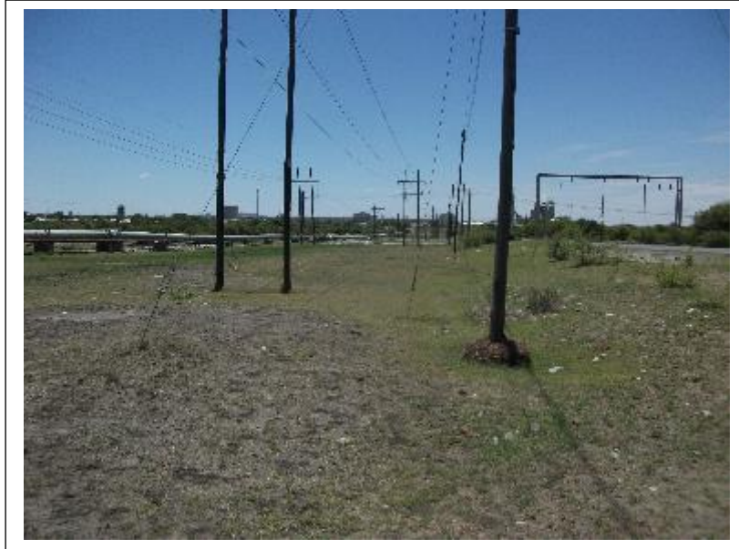
Figure 4- The proposed water pipeline route between the K3 Tailings and the Booster Pump Station already holds a pipeline as well as electric power lines (above).
