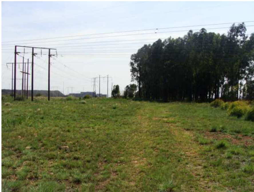
Figure 10 General view along route alternative 3 between industries.
