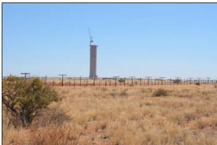
Figure 14. Construction of the neighbouring Khi Solar One CSP Plant
