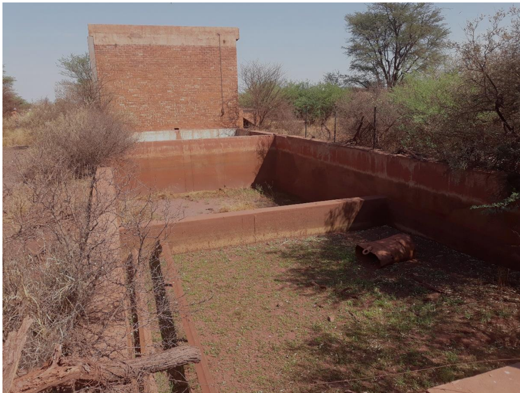
Figs. 26 to 28. Typical views of remaining walls of the settlement tanks. All equipment has been removed and buildings have been vandalised. They have no heritage value. (Photos S.M. Miller 2020.)
