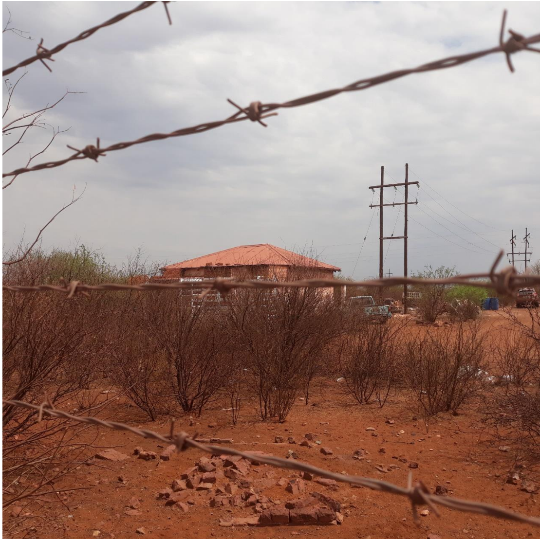
Fig. 23. One of the last inhabited dwellings in Dingleton recorded as “house”. (Photo S.M. Miller 2020.)
