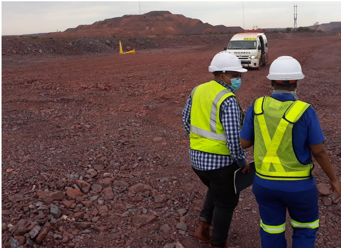
Fig. 17. Work in progress looking west from vp 1. (Photo S.M. Miller 2020.)
