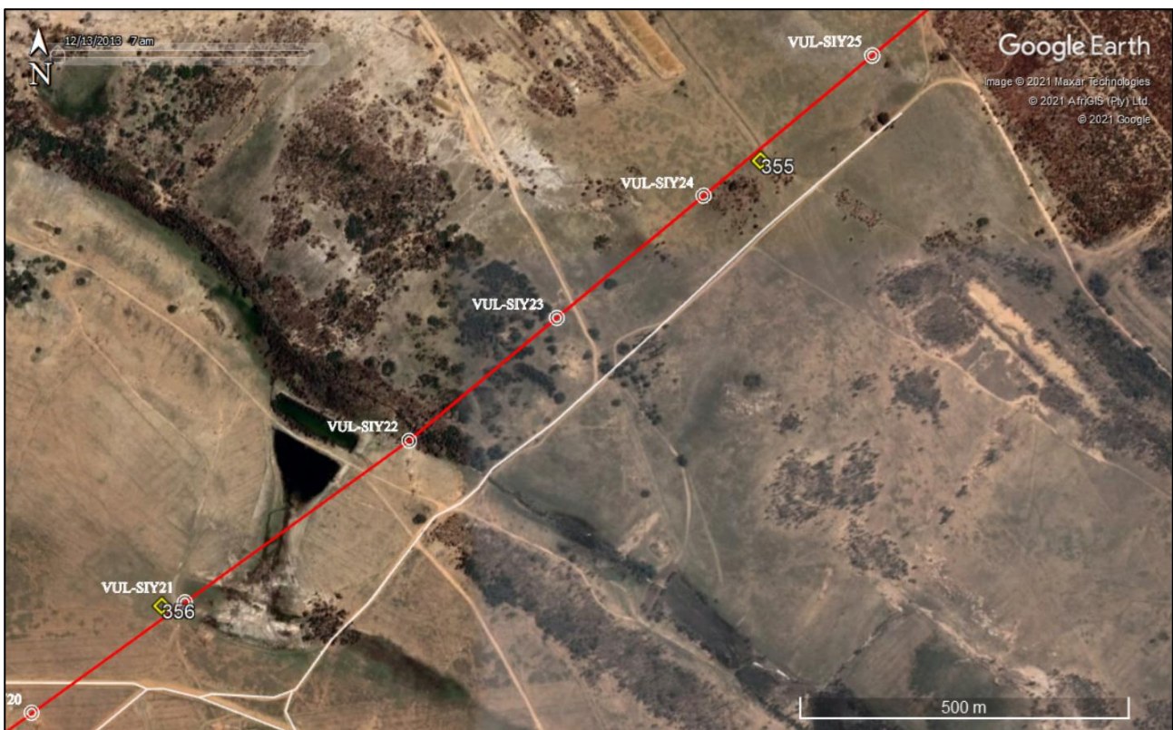
Figure 13: Aerial view of the central part of the study area showing the finds recorded during the survey (numbered yellow waypoints). The pylon positions are shown with white numbered symbols.
