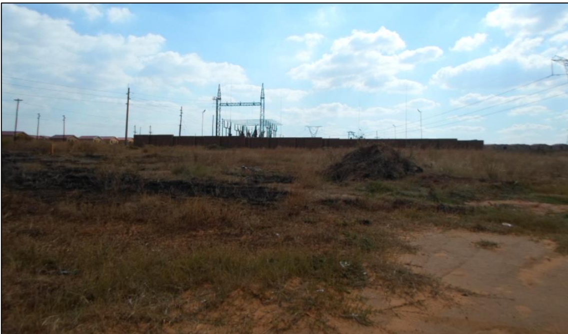
Figure 11: View towards the northwest towards the Siyanqoba Substation with the R544 being towards the left.
