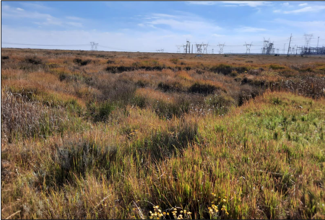
Figure 4: View towards the northwest showing the waterlogged wetland areas to the south of the Vulcan substation.
