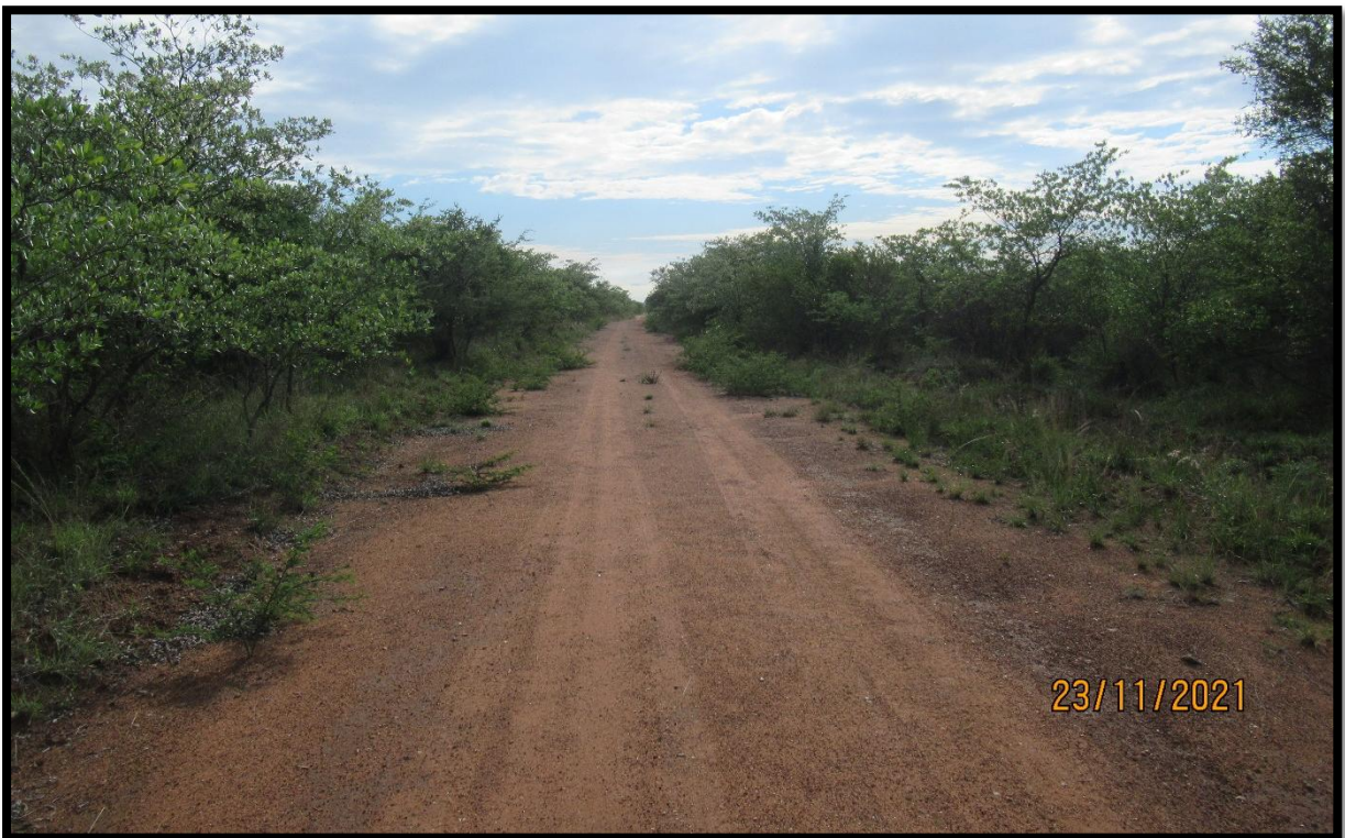
Figure 6: Overall view of the area with road running west-east.
