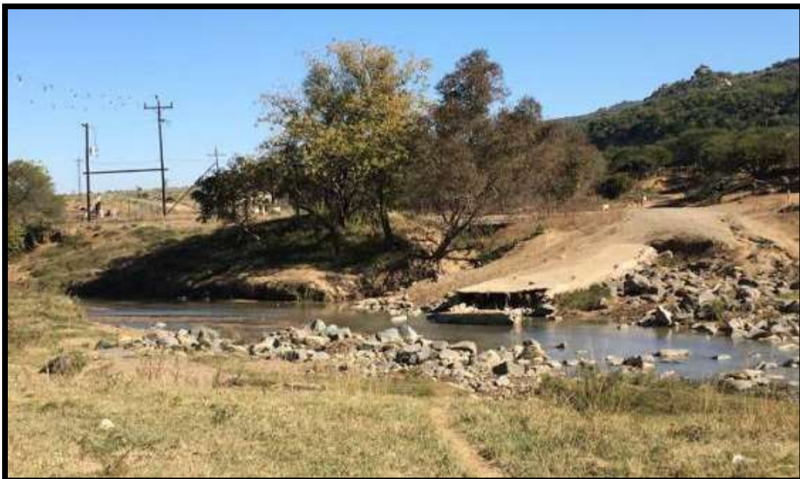
Figure 15. The Madondo Bridge and associated road ,view facing north.
