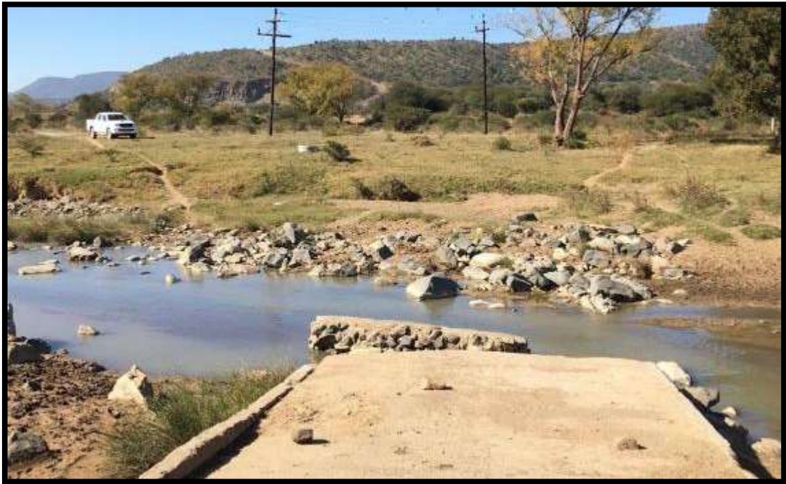
Fig 16. Madondo Bridge, view facing south.
