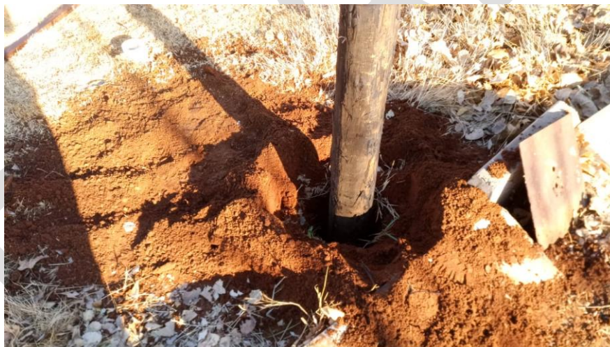
Pole in hole – before backfilling.
