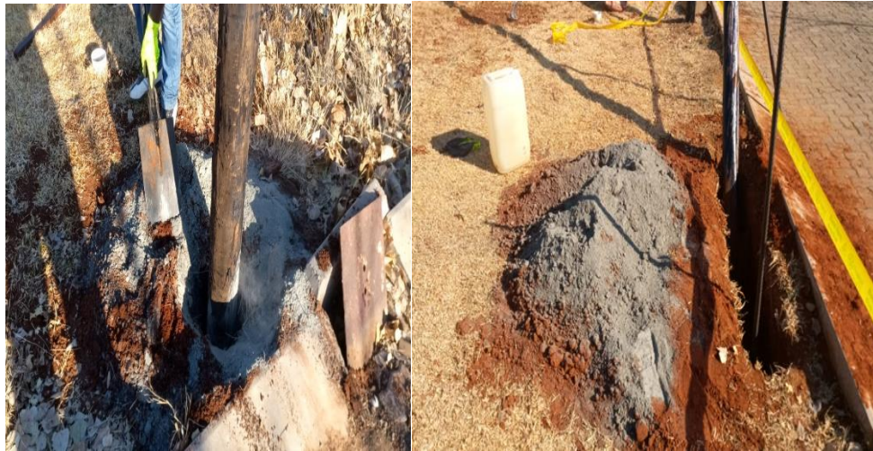
Preparation of Dry mix
