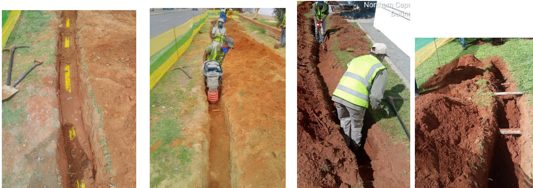
Figures 5 - 8: Some photographs of conventional trenching within the Sol Plaatje Municipal area
