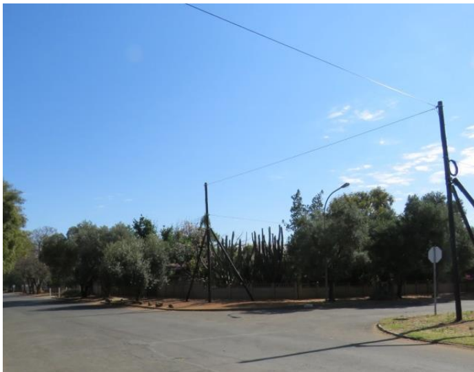
Figure 15: Overhead fibre Hick Street in Sector 1
