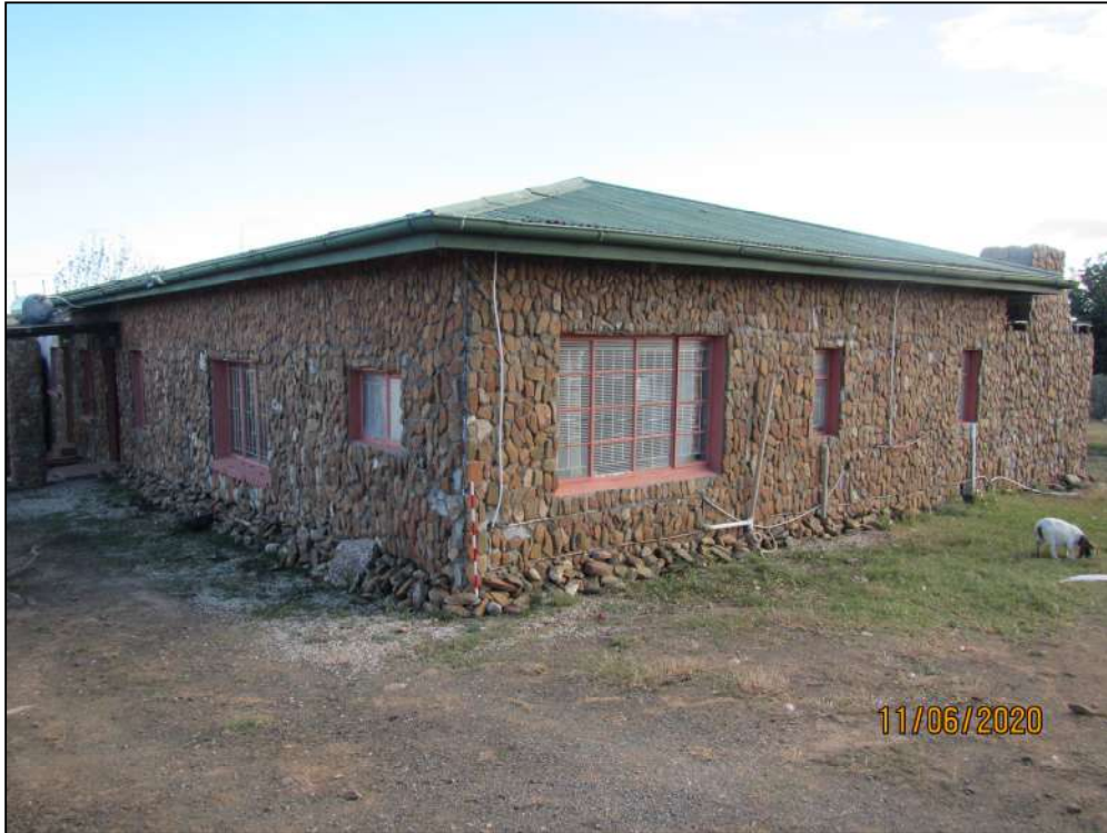
Figure 22 - View of A house, with a stone dressing, was found located on the farm Britzkraal 253 (SF-01). The house is used as overnight accommodation for game hunters.
