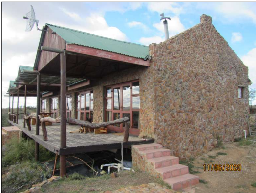
Figure 23 - A house with stone dressing was found on the farm Britzkraal 253 (SF-04). The house is covered in a stone dressing. A low stone wall also surrounds the house.
