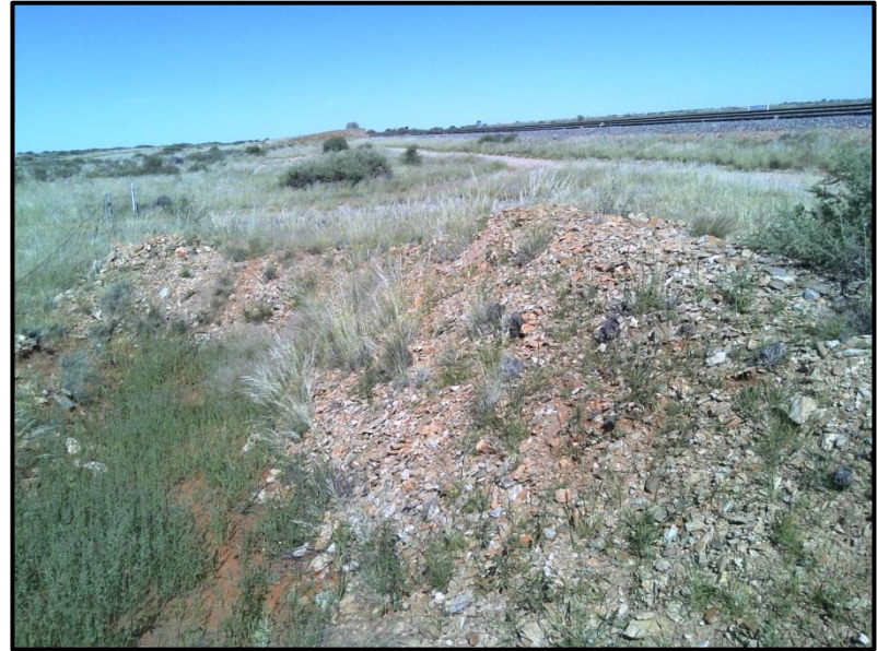
Figure 6. Evidence of earth moving along option 1.
