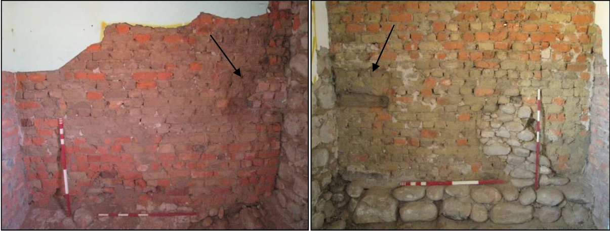
Figure 12: Recess in brickwork of wall 269, Area 2, view to north
