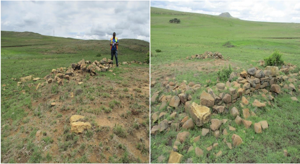
Figure 11: View of the collapsed stone walling in the proposed area.
