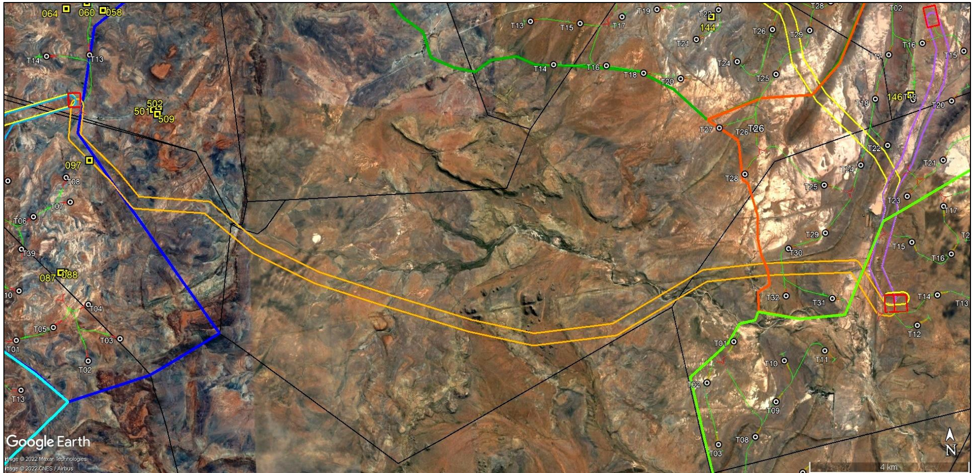
Figure A1.7: GoogleEarth© satellite image showing the 300m wide 400 kV powerline corridor (orange) connecting the Taibos collector substation in the west and the Soutrivier collector substation in the east (red rectangles). Fossil site Loc. 097 refers to scrappy plant remains of low scientific and conservation value for which no mitigation is recommended. Very little time was spent within the 400 kV powerline corridor during the reconnaissance-level site visits so a pre-construction palaeontological walkdown of the authorised powerline footprint here is essential.
