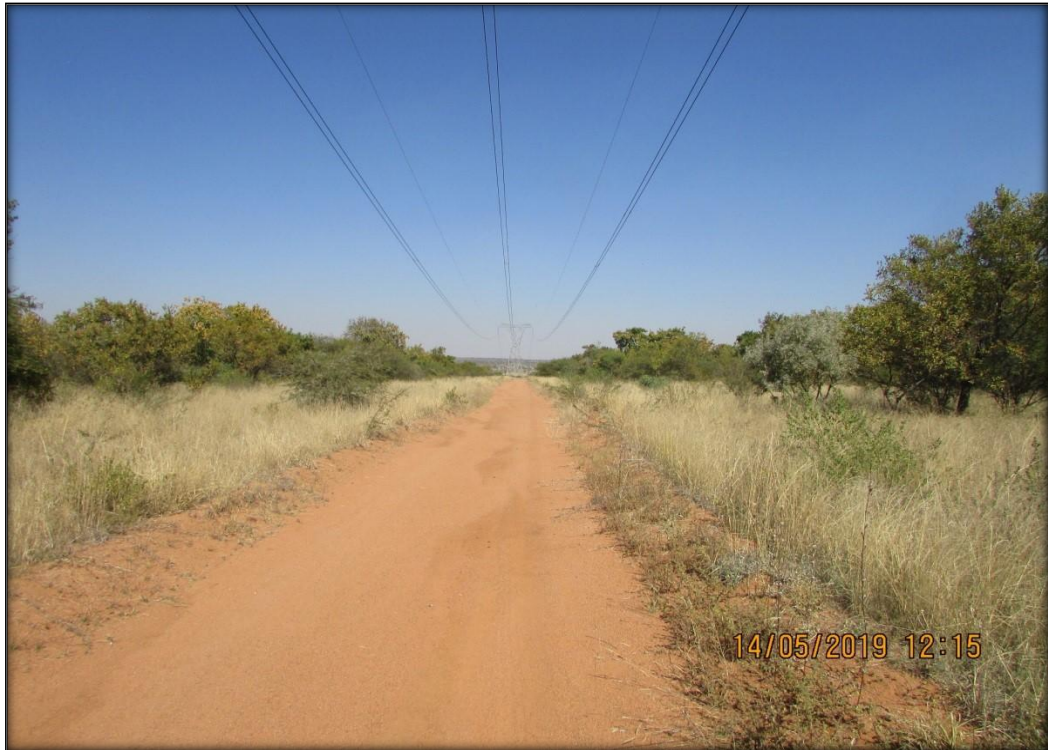
Figure 6: View down Eskom Power Line corridor.
