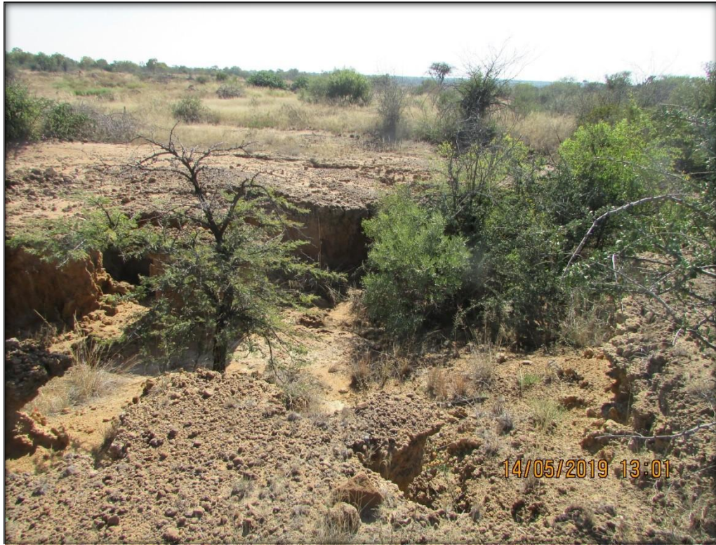
Figure 14: Another view of Site 1.
