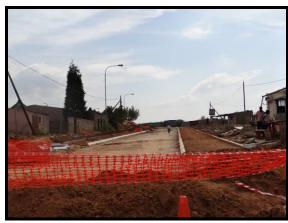
Construction of new tar road with paving on both sides of the road
