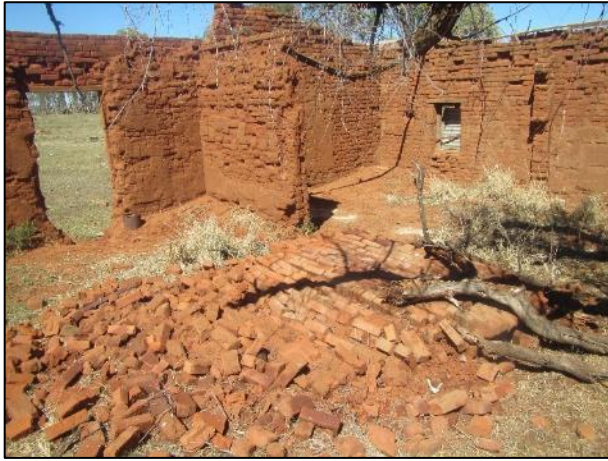
Figure 22: Interior of the brick house at waypoint 295.
