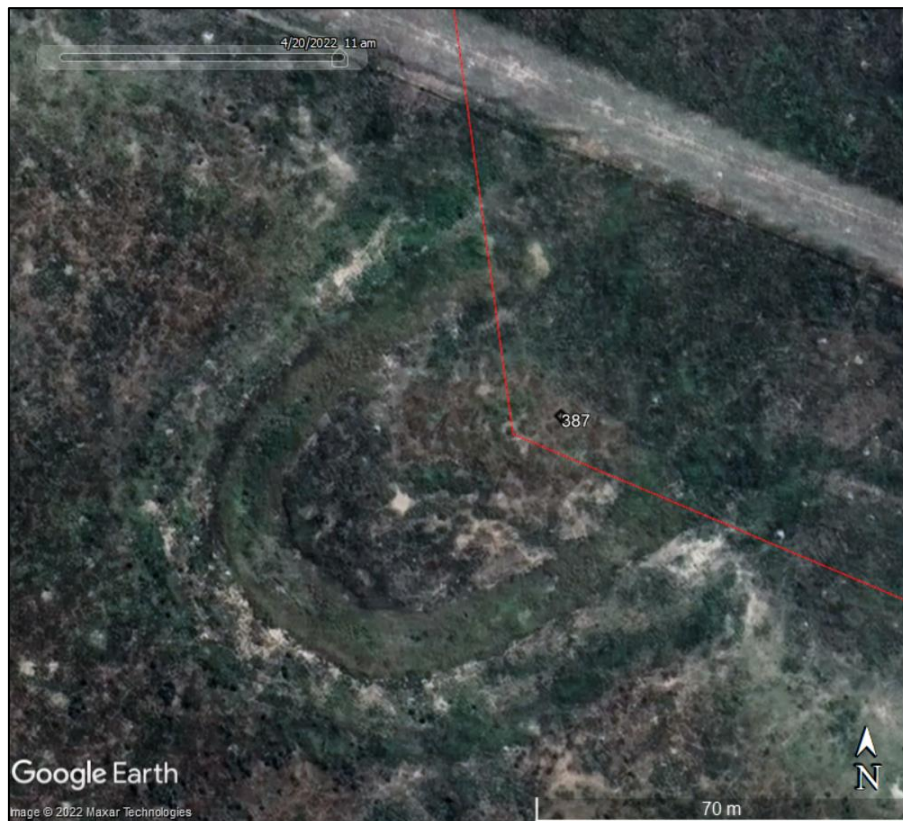
Figure 15: Aerial view of the earthen dam at waypoint 387.
