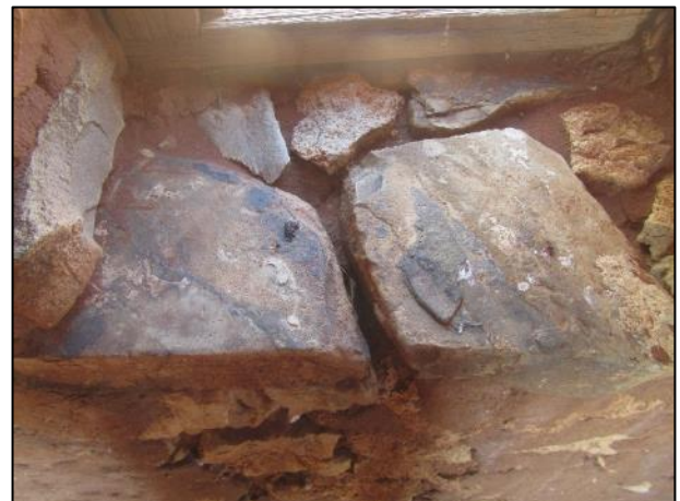
Figure 19: Windowsill in the cottage at waypoint 294.
