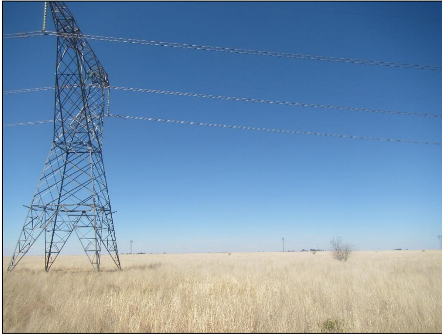
Figure 6: View towards the east in the north-western part of the corridor.
