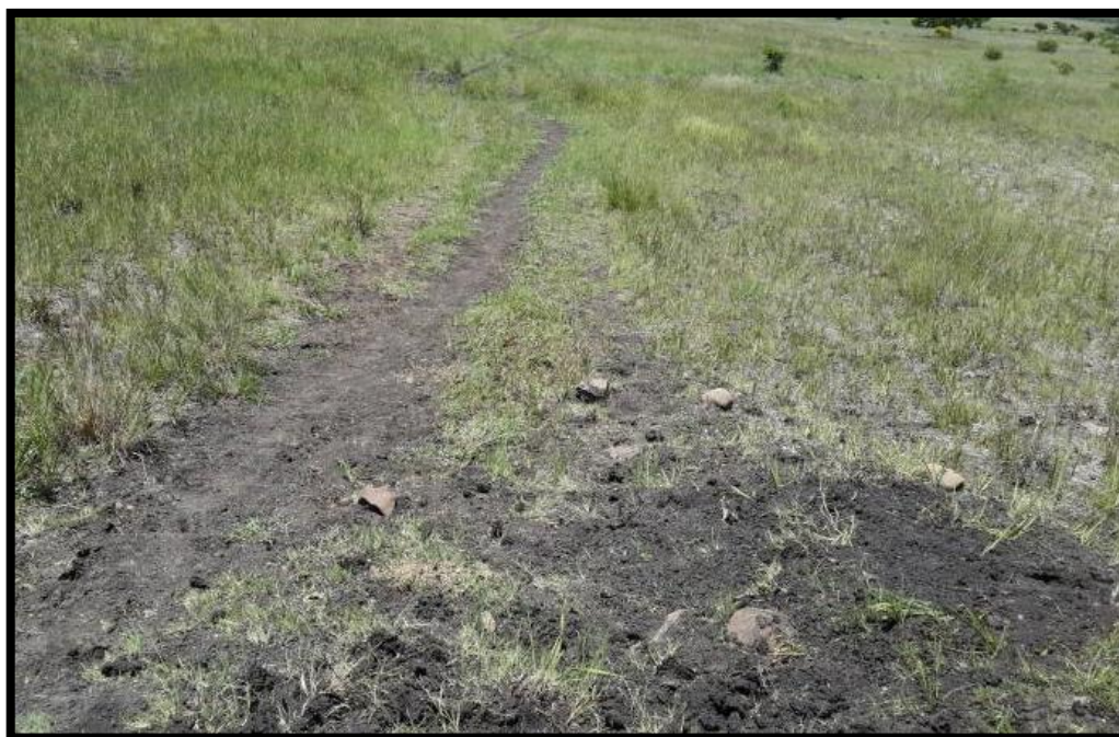
Figure 4. The proposed Squbudu Extension Road that has been earmarked for upgrading.
