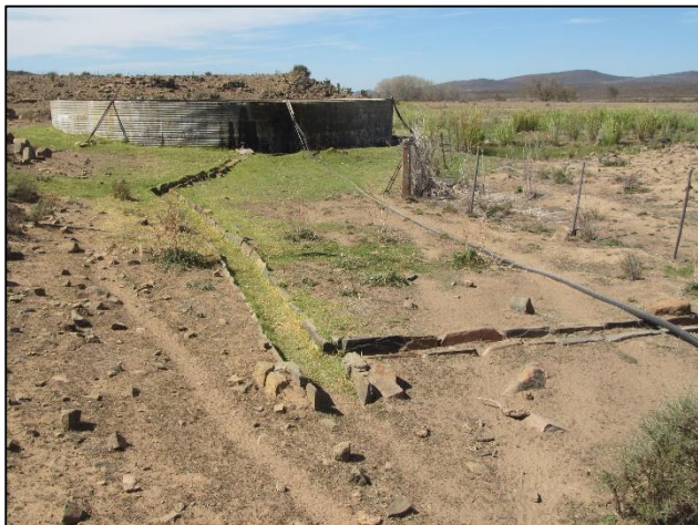
Figure A5.3: The cement dam and stone-lined water furrows at waypoint 097.
