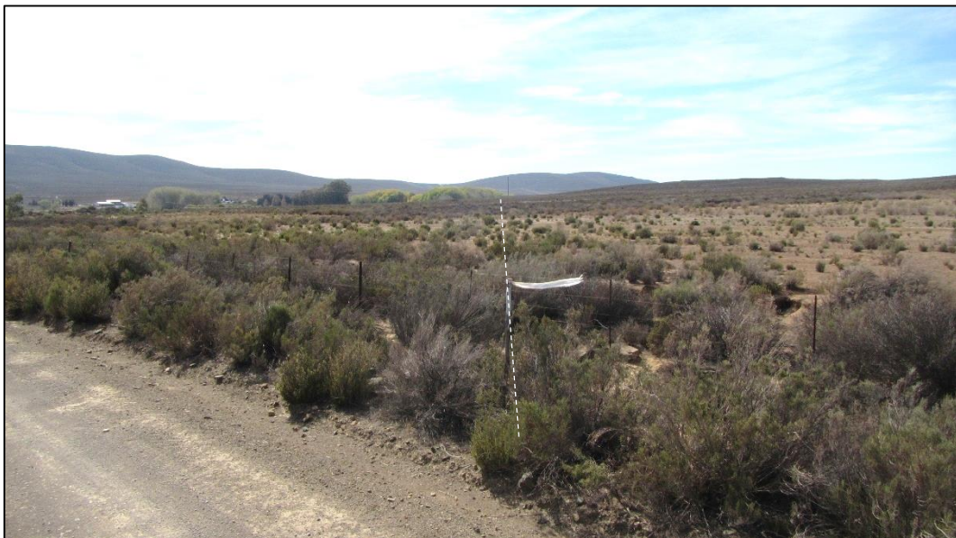
Figure 4: Looking towards the northeast along the western-most section of the new road alignment (white dashed line) where it leaves the main gravel road.
