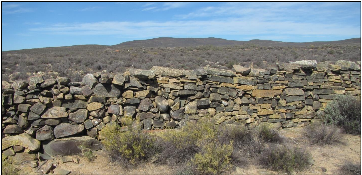
Figure 16: View of the wall at a section where the type of rock used changes from rounded and sub-angular rocks to slabs (waypoint 082).
