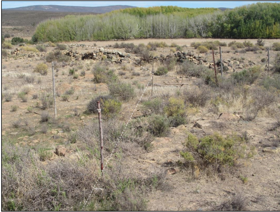
Figure 25: View towards the southwest along the originally proposed road alignment (white dashed line). The alternative alignment that will be implemented lies out of view just to the right.
