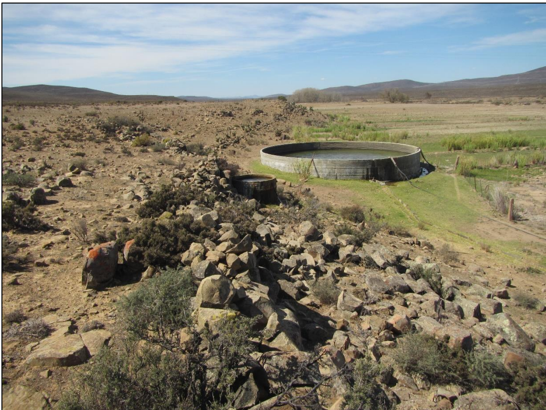
View towards the east along the edge of the river floodplain at waypoint 098 showing the light stone walling running along the top of the low cliff line.
