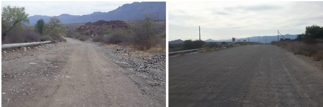
Figure 7: Existing roads in the surveyed area.
