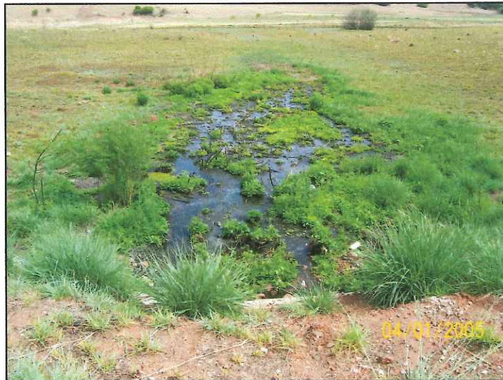
Fig 28: Effluent from the multiple septic tank system at Sterkfontein caves spills over into the Blaauwbank River, an already heavily polluted drainage system. The throughput at Sterkfontein exceeds design specifications and an upgrade is planned. The overflow seen here is on its way to the Blaauwbank at the valley bottom seen in the distance
