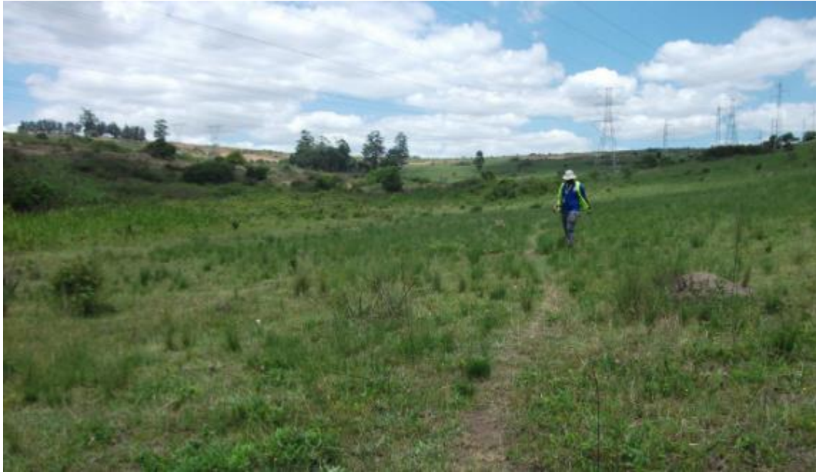
Figure 9: Pipeline route looking towards the west
