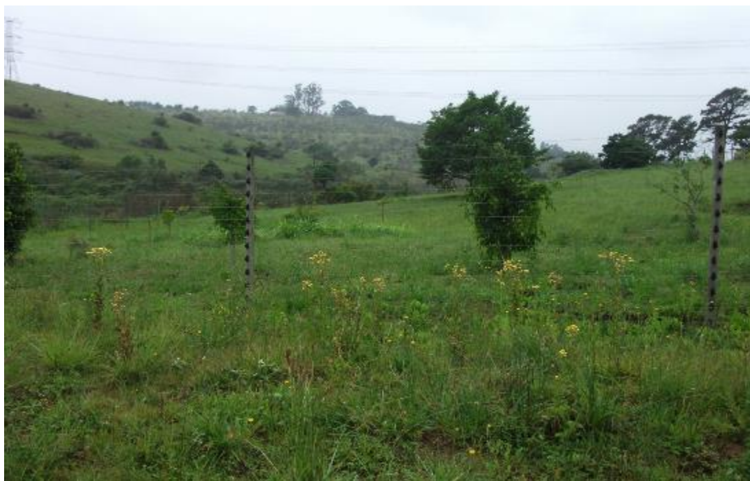
Figure 15: Section of pipeline situated on privately owned land
