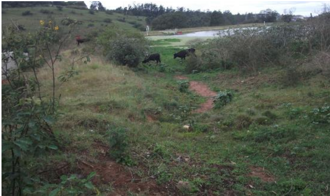
Figure 8: Dam with fencing in left hand corner
