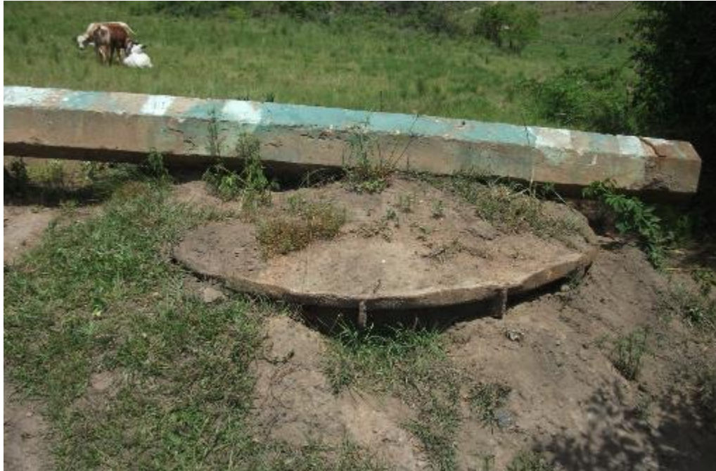
Figure 11: Possible stormwater infrastructure
