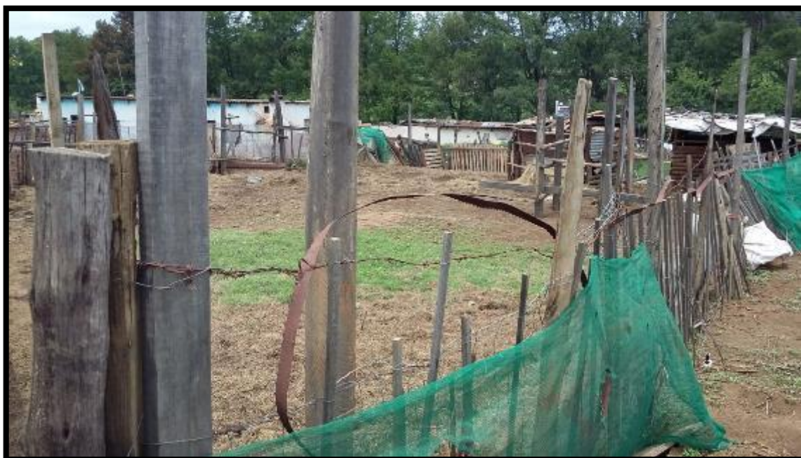
Figure 13. Shacks and associated structures: no heritage value.
