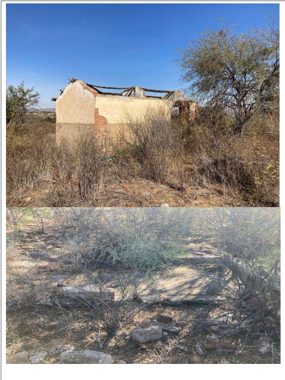
Figure 11: Old settlement: abandoned farmhouse.
