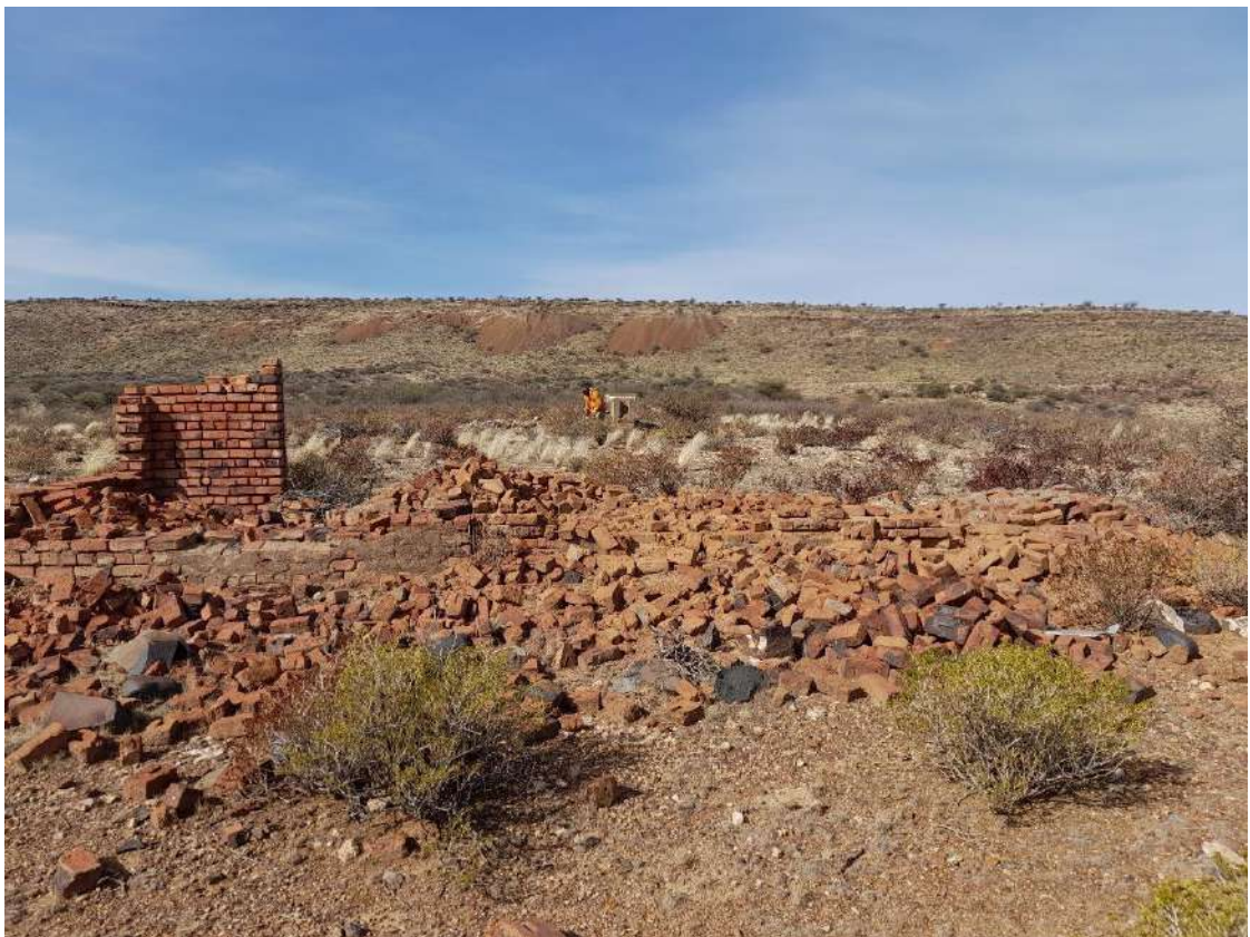
Figure 20: collapsed brick structure, with old mine tailings in the background
