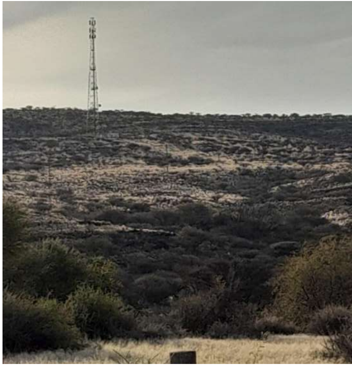
Figure 35 : Telecommunications mast indicating current land use
