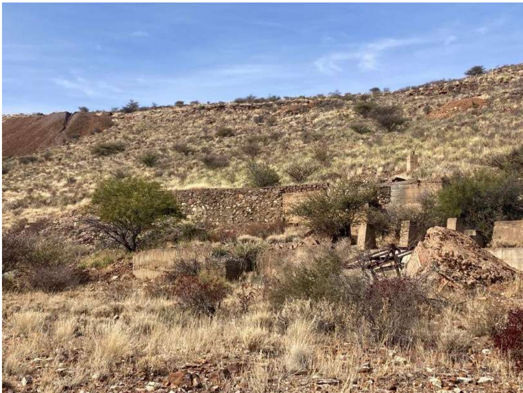
Figure 32: Abandoned ore loading infrastructure, with tailings in the background and crocidolite on the surface.
