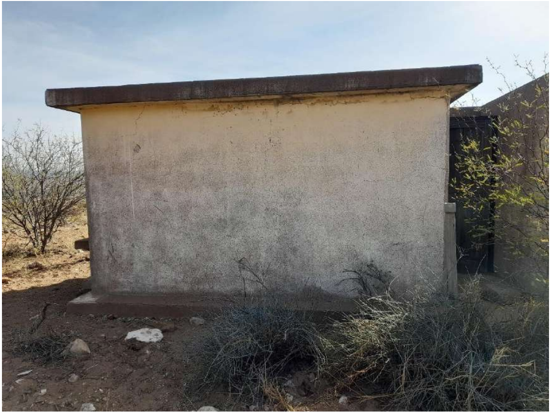
Figure 19: storehouse of dangerous chemicals and explosives, several foundations
