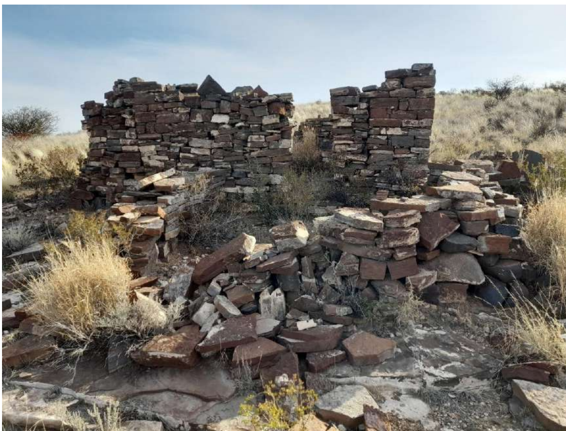
Figure 23: House structure constructed in banded iron stone blocks
