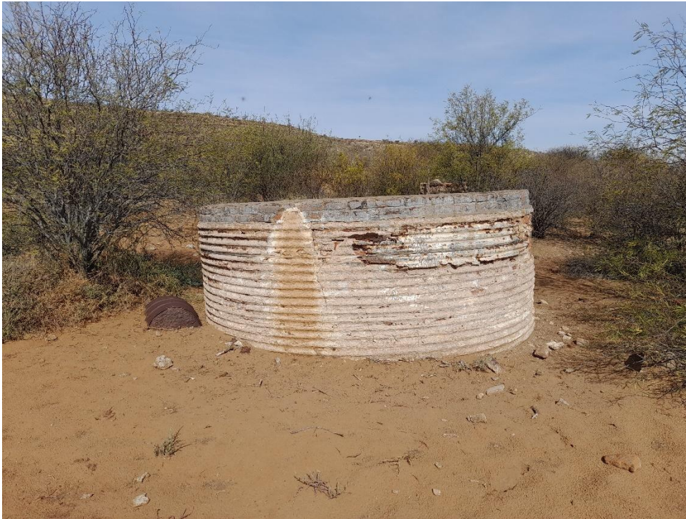
Fig 9: Abandoned explosives room possibly for mining activities on label S7. Next to the explosives room is abandoned animal watering infrastructure (tank, drinking trough) and abandoned stone structure.
