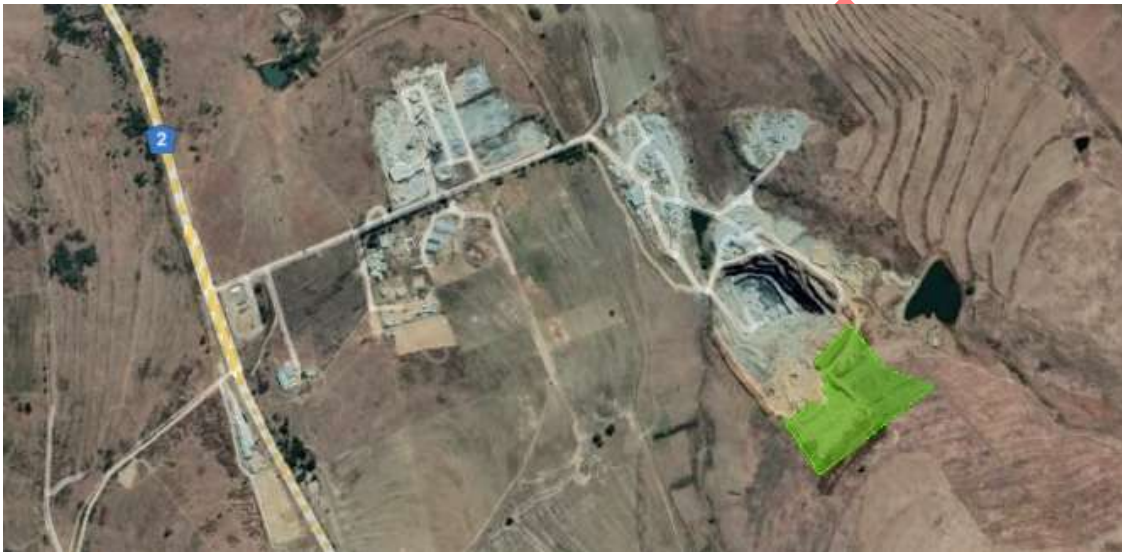
Figure 1: Location of the Stonewall quarry and extension (green). The image source is Umlando & GoogleEarth).
