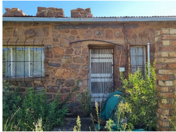
Figure 9: Main farm building indicating different modification and alterations. In left image, note abutting wall joint, illustrating different phases of modification.
