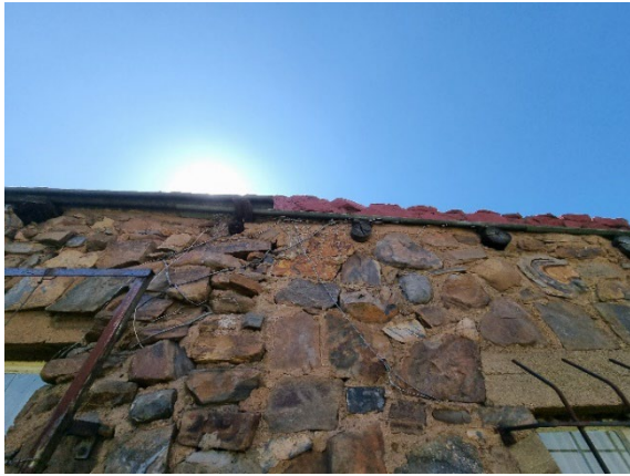
Figure 9: Main farm building indicating different modification and alterations. In left image, note abutting wall joint, illustrating different phases of modification.
