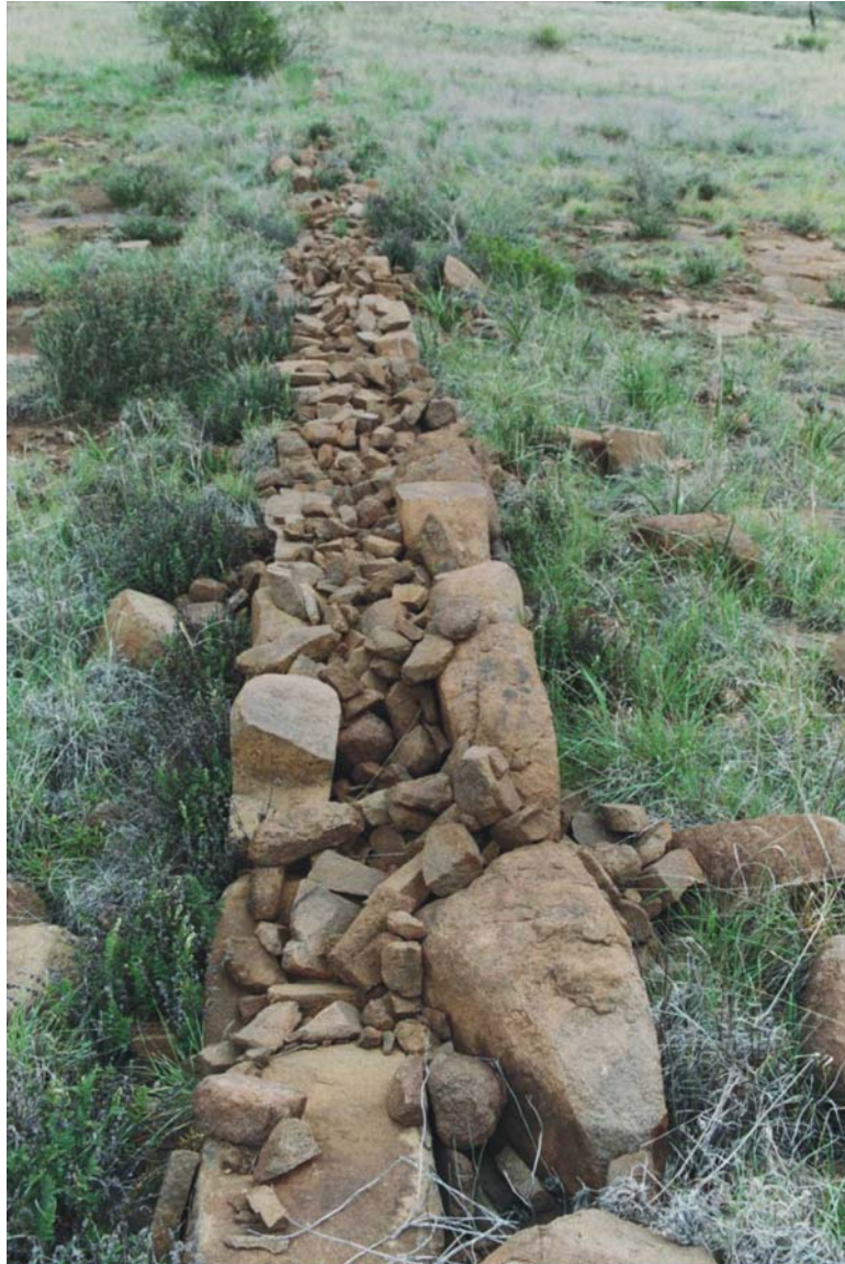
Figure 28: Construction of the wall showing large boulders on the outside with smaller rocks on the inside
