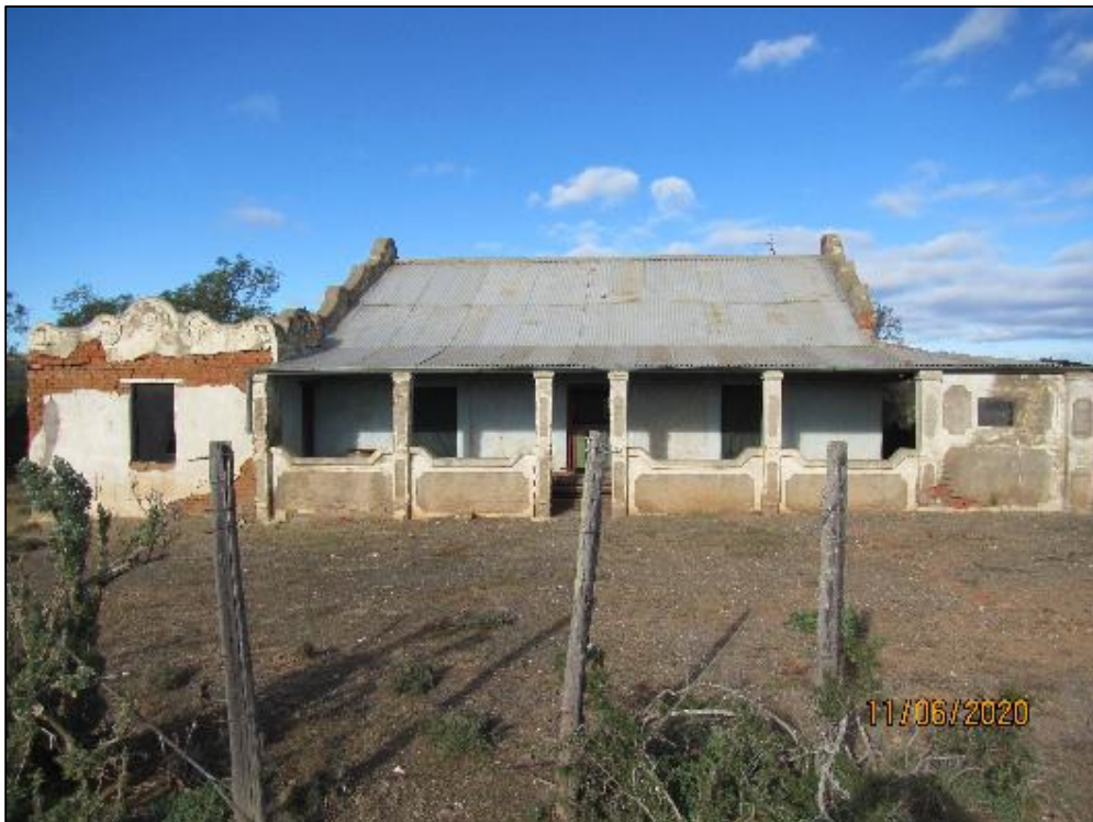
Figure 25 - A dilapidated house with a small outbuilding was found on the farm Britzkraal 253.
