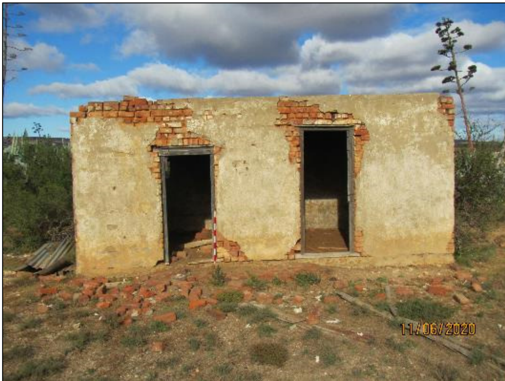
Figure 31 - A dilapidated brick labourer house was found on the farm Britzkraal 253 (SF-09). The windows and doors of the house have been removed, and the house has been abandoned.
