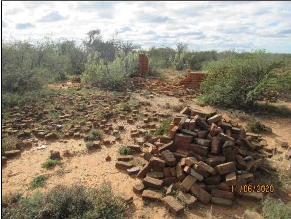
Figure 32 -A ruined brick labourer house was found on the farm Britzkraal 253 (SF-10). The windows and doors of the house have been removed, and the house has been abandoned.
