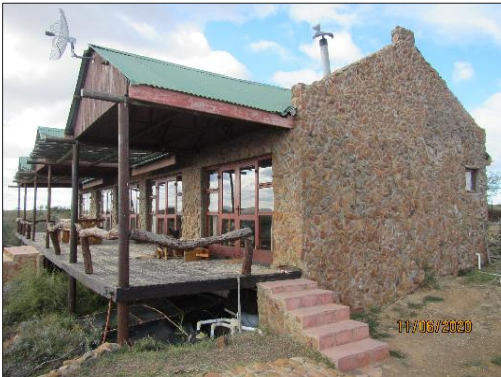
Figure 23 - A house with stone dressing was found on the farm Britzkraal 253 (SF-04). The house is covered in a stone dressing. A low stone wall also surround the house.
