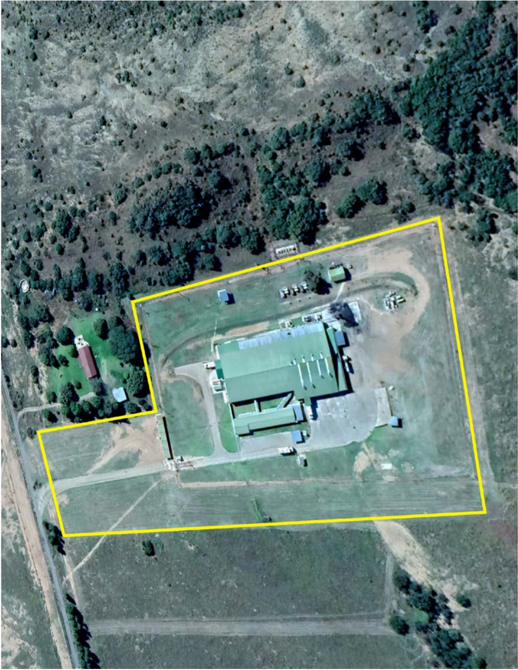
Figure 3. Aerial view of poultry processing facility at Boesmanskop.
