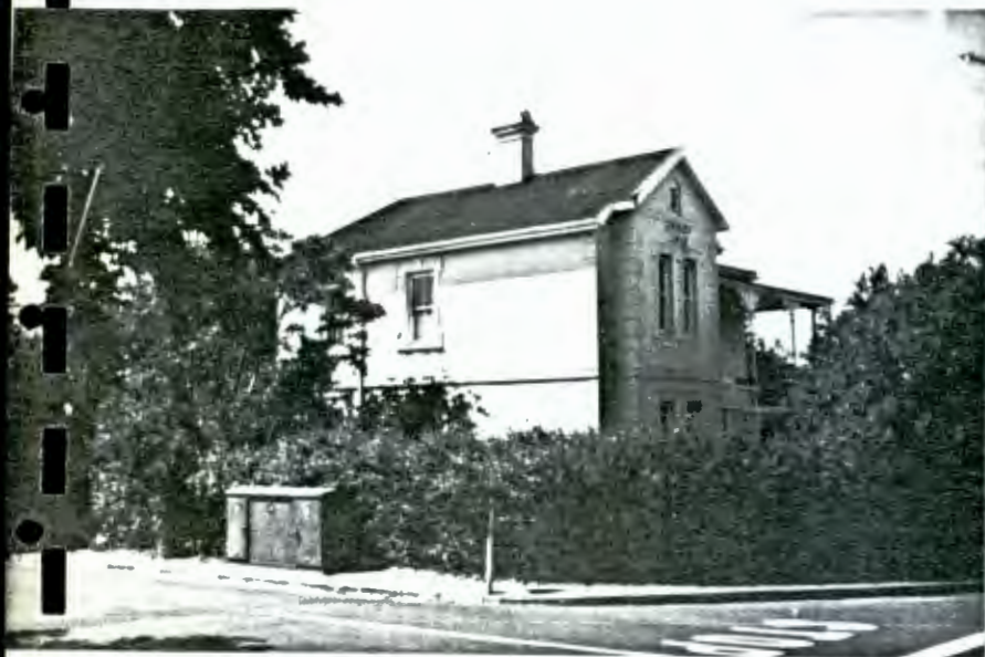
27 Church Street, Durbanville
