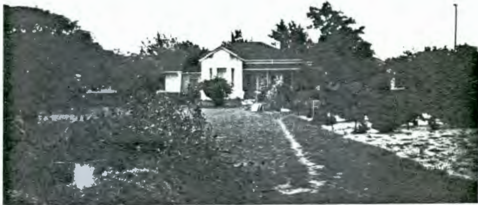
20 Church Street, Durbanville
