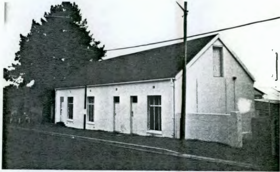
(prob.) No. 8 Gladstone Street, Durbanville
