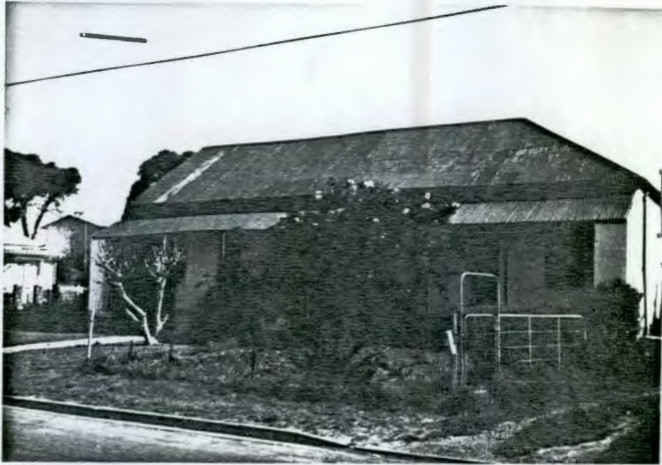
Semi-detached house, Gladstone Str. c/o Queen Street, Durbanville
