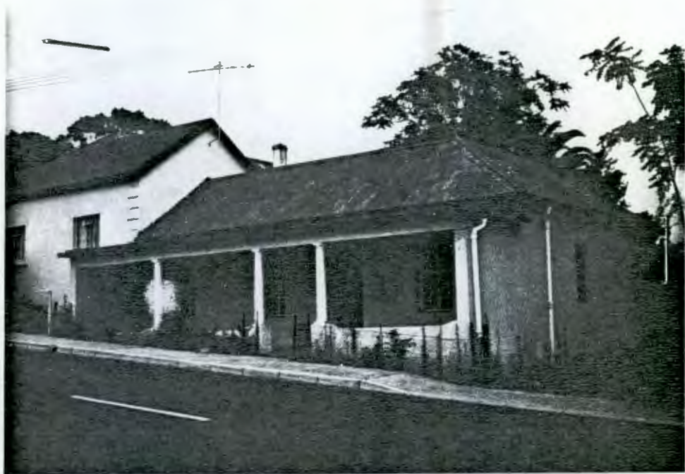
7 Upper Church Street, Durbanville
