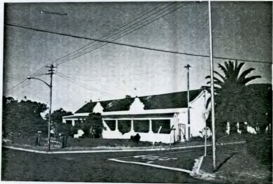
Semi-detached house, 12 Queen Street c/o Gladstone Str., Durbanville
