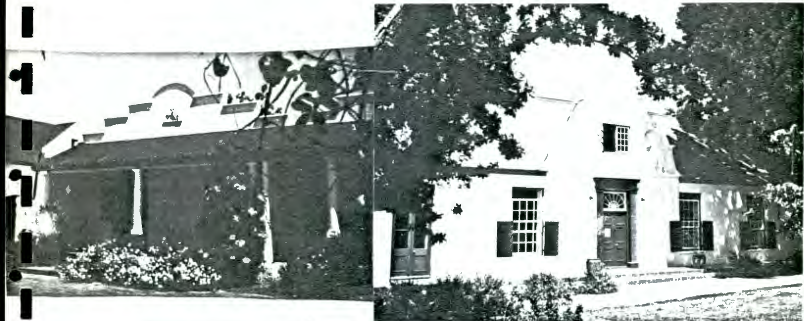
RUST-EN-VREDE (Meneely House), Wellington Rd, Durbanville
