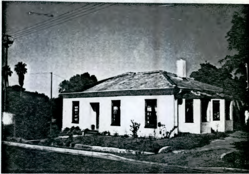
HOUSE AND CHAPEL, 32 Queen Street, Durbanville
