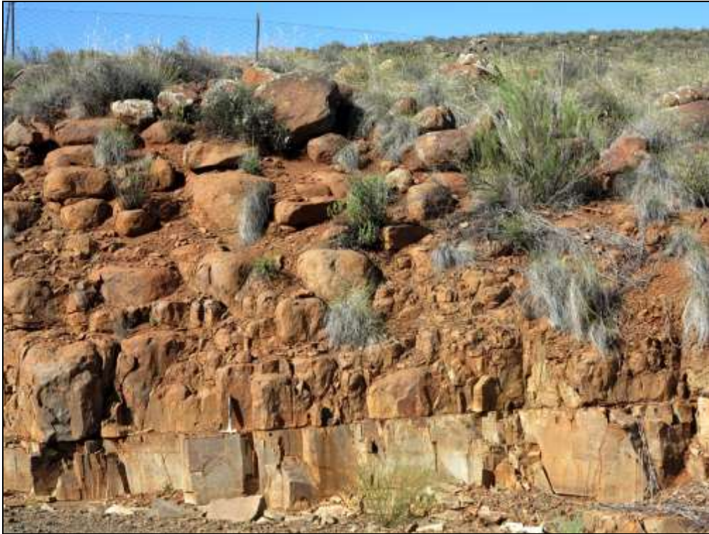
Fig. 5. R354 road cutting through the massive sill at Rooikloof showing the sharp lower contact with baked channel sandstones of the Abrahamskraal Formation as well as typical rusty-brown lateritic and corestone weathering of the dolerite body itself (Hammer = 30 cm).
