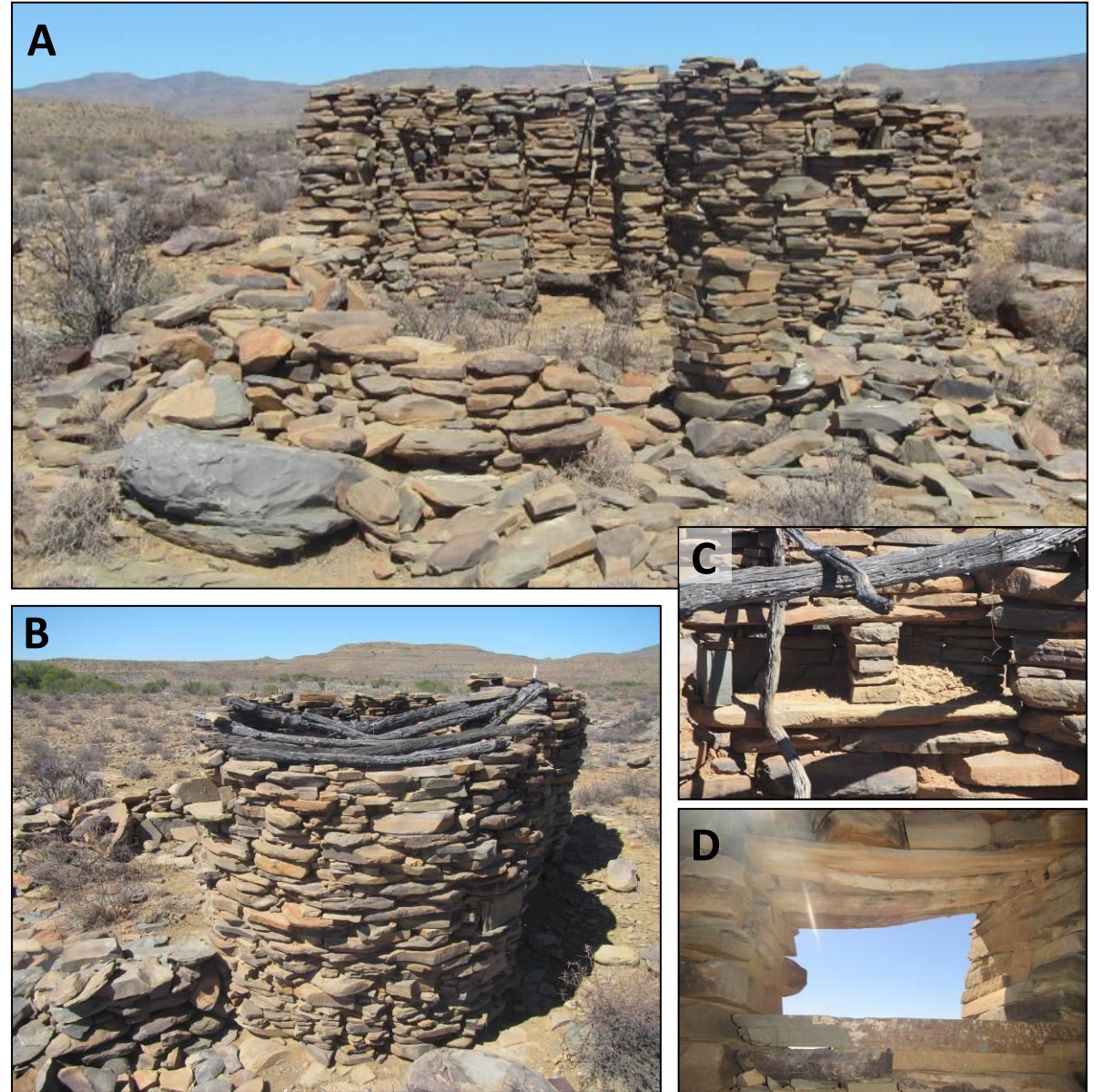
Figure 33: Plan of the ruined stone-walled house at waypoint 500 with (A) a view towards the west of the entrance, (B) a view towards the south of the northern lobe showing remaining roof 'beams', (C) a view of the high 'muurkas' in the western lobe and (D) a view of the east-facing window with wooden planks and sticks in the southern lobe. Not to scale but approximate measurements are indicated.
