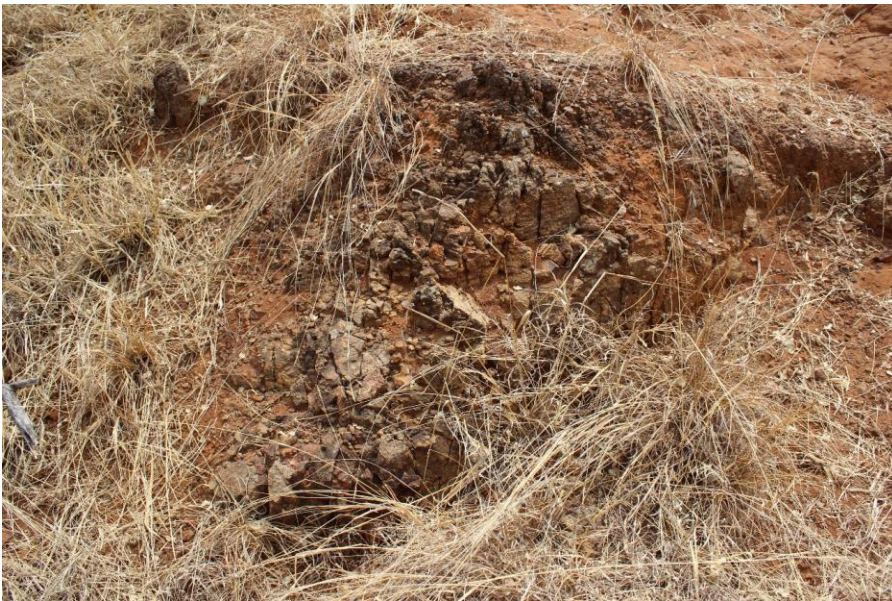
Figure 6- Traces of quarry wall from previous road construction or rehabilitation activities
