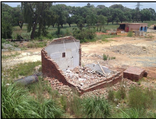
Figure 35: Demolished structure on site
