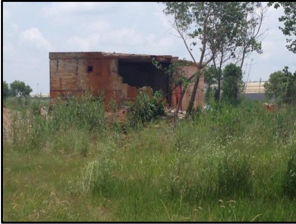
Figure 29. Demolished structure on site
