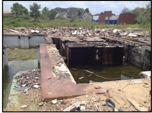
Figure 38: Demolished structures on site.
