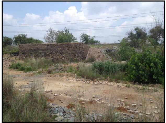
Figure 32. Demolished structure on site
