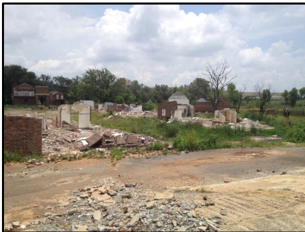
Figure 39: Demolished structures on site
