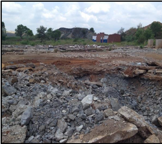
Figure 31. Demolished structure on site .
