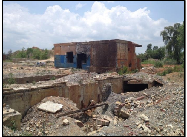
Figure 30. Demolished structure on site
