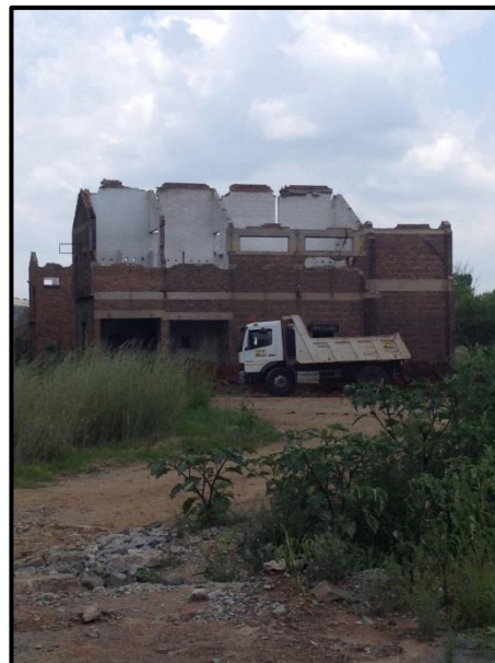
Figure 40: Demolished structure on site.
