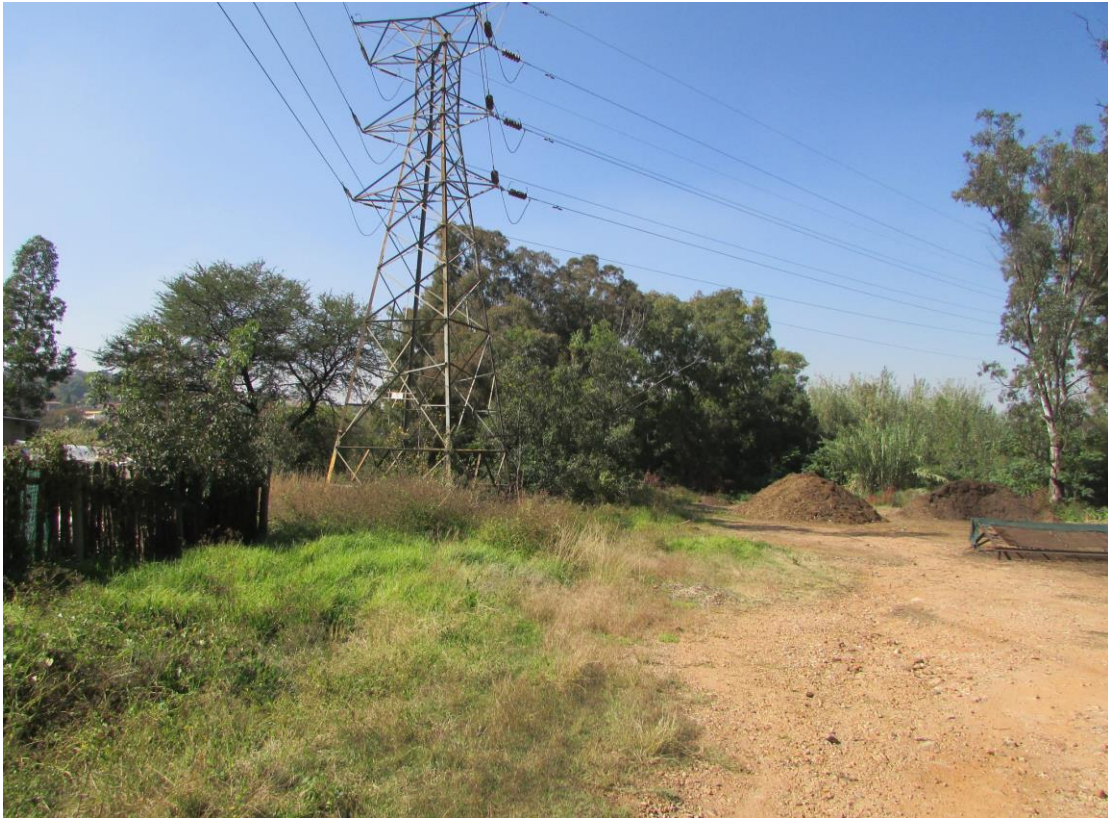
Figure 12: A view of the existing Powerline that will be utilized as well.
