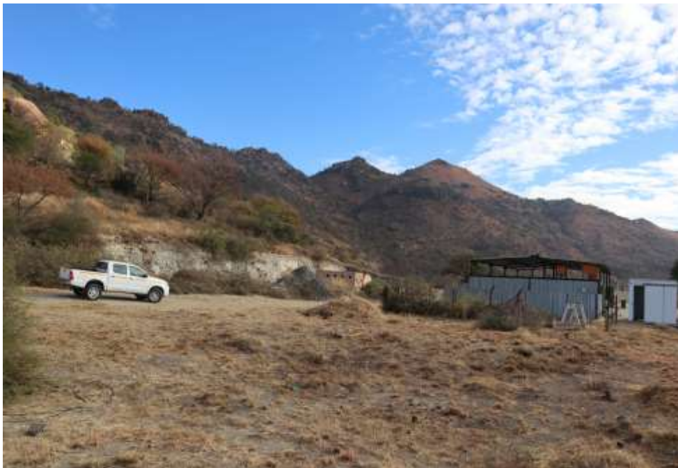
Figure 9: General view of Merensky Shaft.
