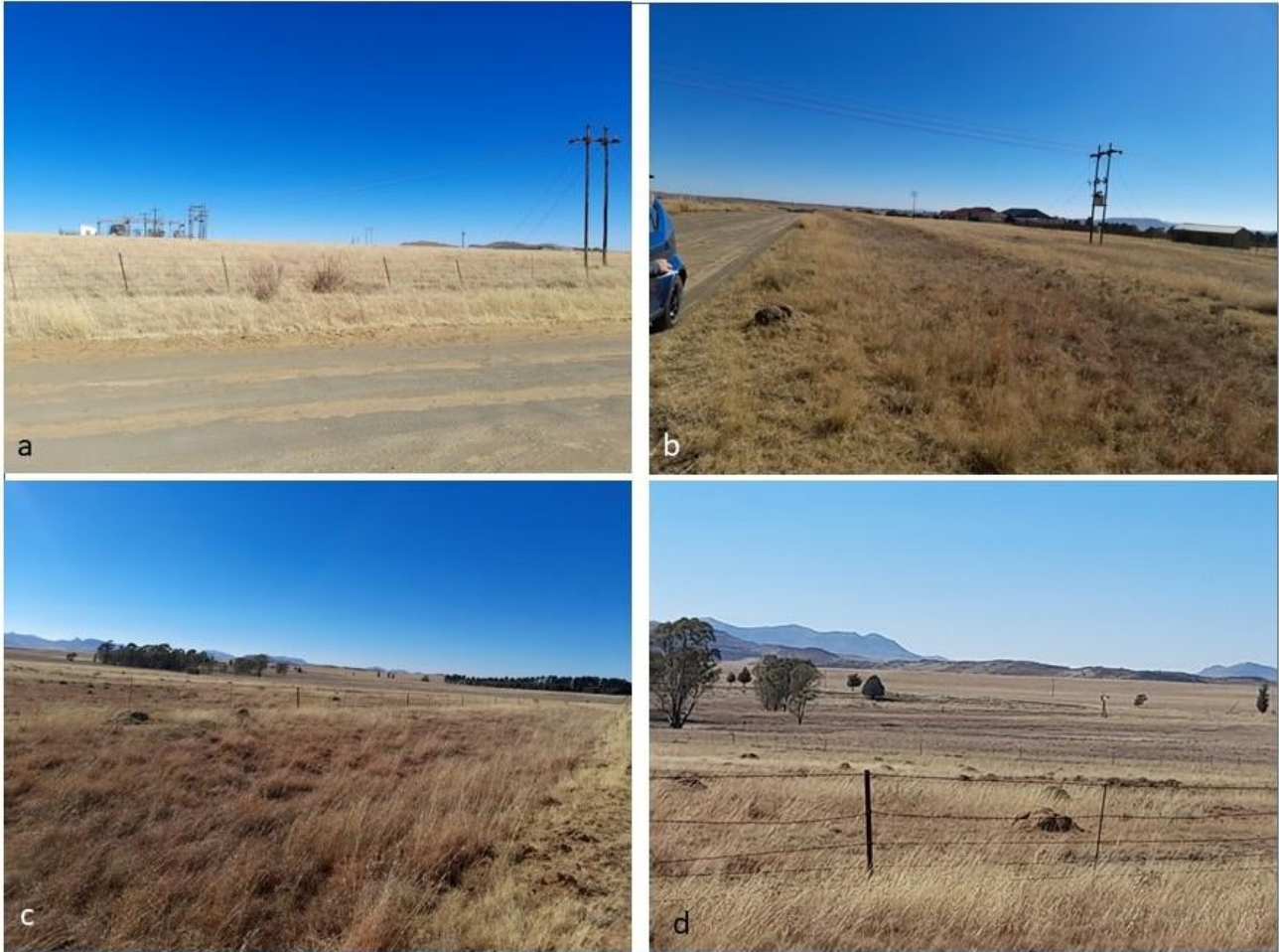
Figure 5: Rouxville (to Smithfield) Stop 11; a – existing Rouxville substation with powerline leading in; b – powerline leading northwards towards Zastron; grassland vegetation along powerline route close to the substation; c – grassland vegetation along powerline route; d – grassland along route farther along.
